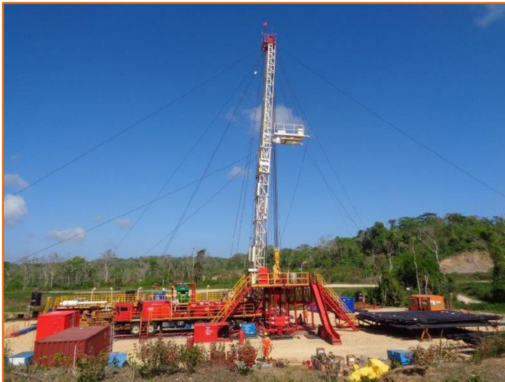
Drilling operations at the Morne Diablo field
