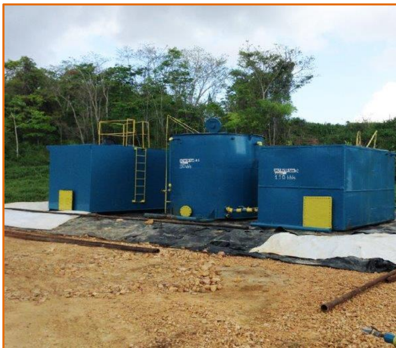
Waterflood operations at Morne Diablo field
